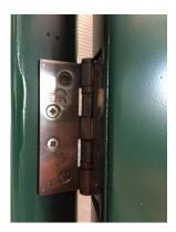
Reveal fix butt hinges are supplied ready lubricated by the manufacturer to ensure smooth operation of hinge leaves when fitted to doors. In some cases, after installation there will be signs to varying degrees of clear oil seepage. If left for a period and particularly in high usage areas the oil will combine with atmospheric dust and
