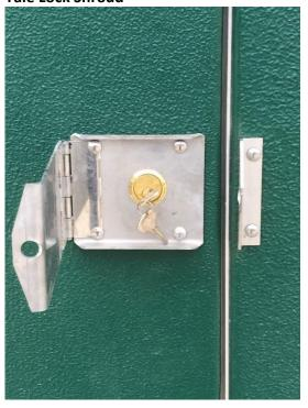
This is bolted to the door and should require very little maintenance apart from checking they are secured tightly to the doors and tightened if required.
