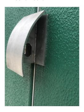
Door shrouds are bolted to the doors and act as an additional security measure as an additional padlocking point and to protect padlocks or handles from vandalism.
