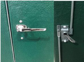
These mechanisms are bolted to the opening door leaf and should require very little maintenance apart from regular cleaning / lubricating.
